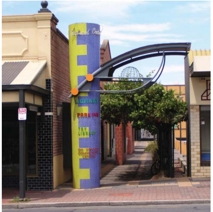
Existing Signage Pillar
